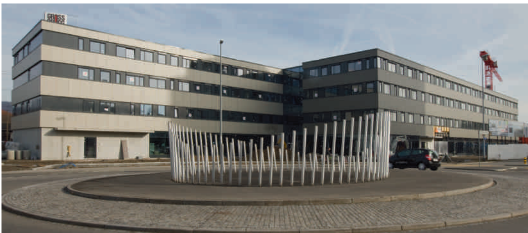
Gais Center in Aarau
